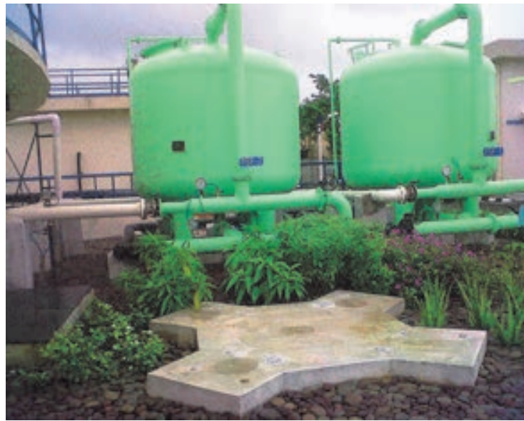
Pressure Sand Filters
